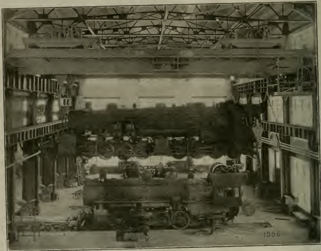
HEAVIEST TYPE LOCOMOTIVE CARRIED OVER ANOTHER LOCOMOTIVE BY THE USE OF A POWERFUL SHOP TRAVELING CRANE.
